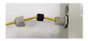
**Step 2:** Push the rubber gasket into the threaded cable guide, then screw the weather shield cap over the threaded cable guide to seal the cable opening.
